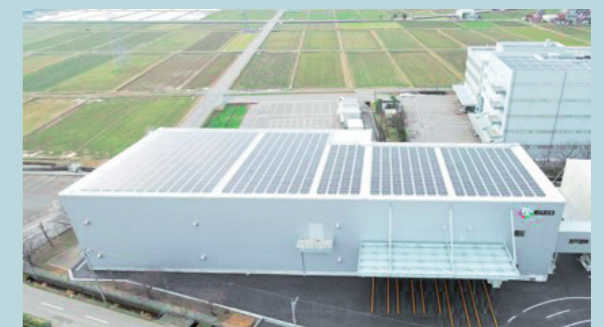
EIZO Corporation Logistics Building (Japan, FY2022)
